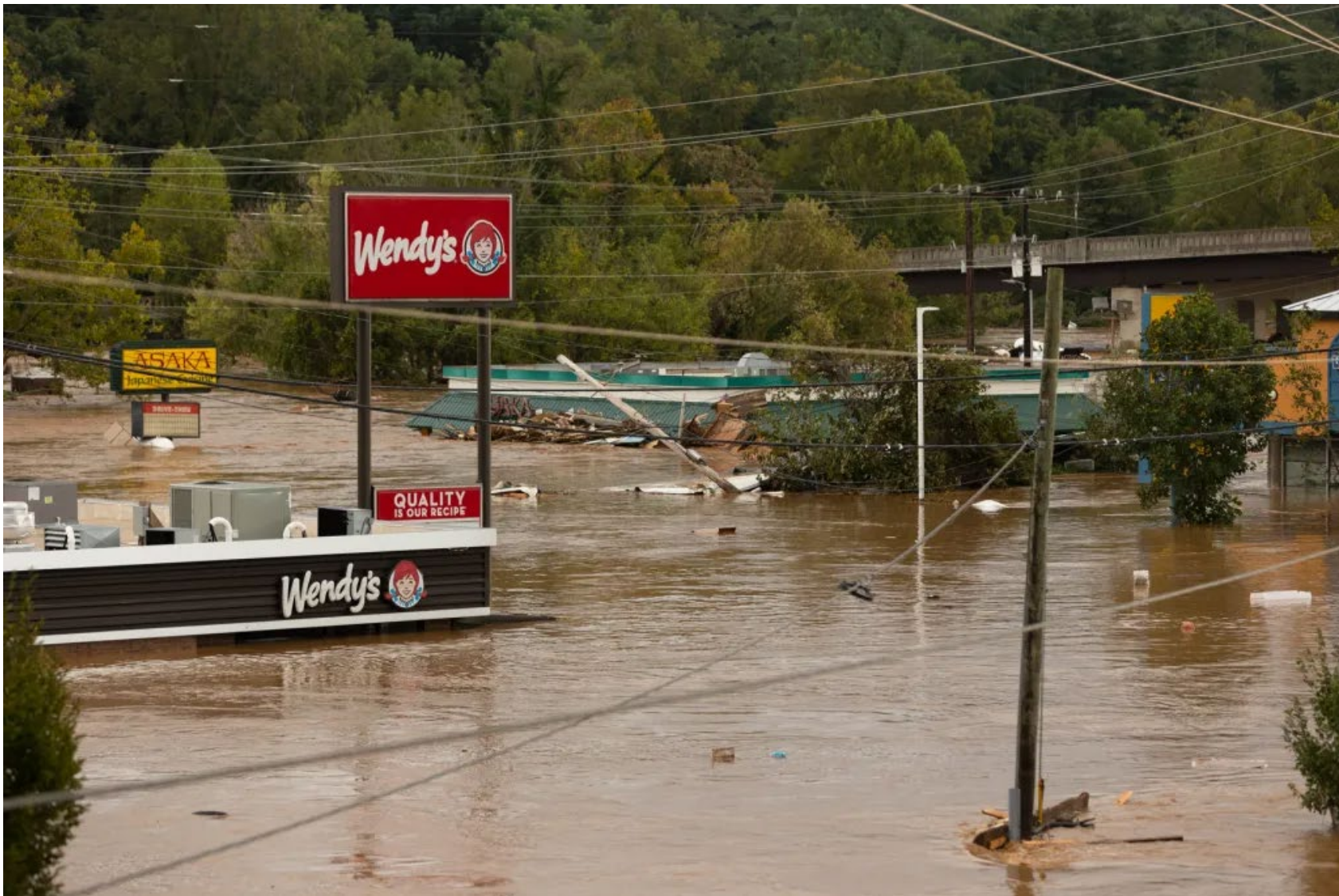
Figure 29. Flooding from the Swannanoa and French Broad rivers in Biltmore Village in Asheville, NC after Helene swept through on 27 September 2024. Image courtesy of Colby Rabon and the Carolina Public Press.
