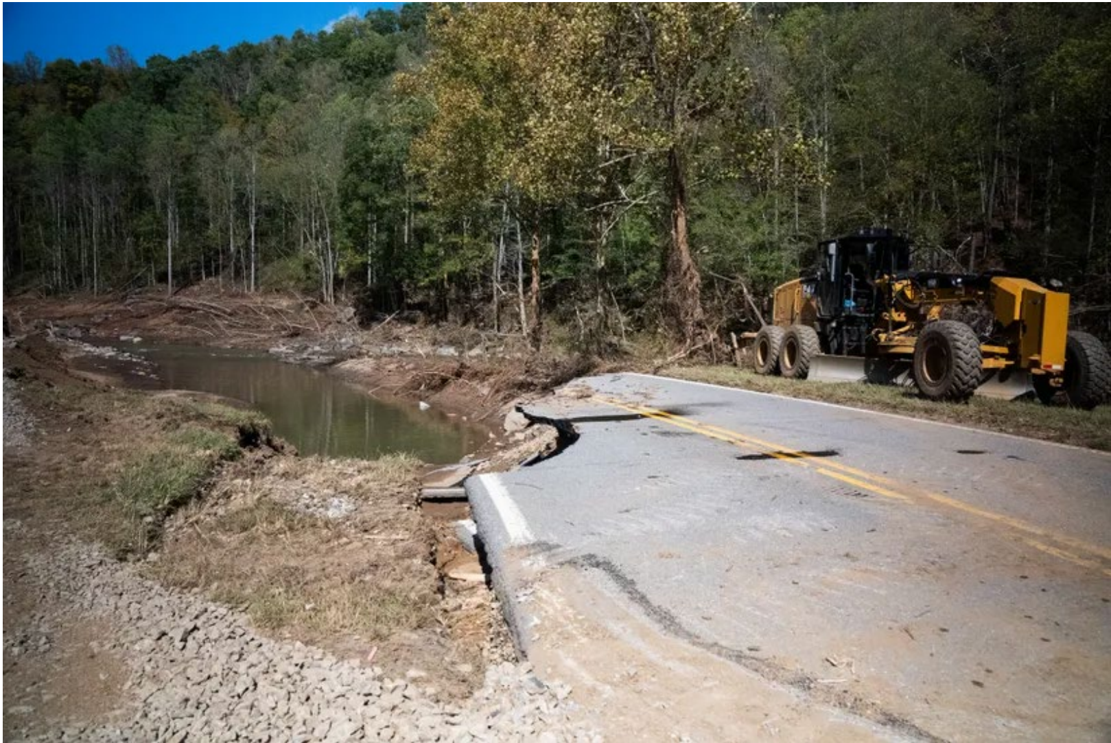
Figure 34. U.S. Route 19 in Yancey County is just one example of hundreds of roads that were washed out and destroyed in western North Carolina. Photo courtesy of Josh Morgan and USA Today.
